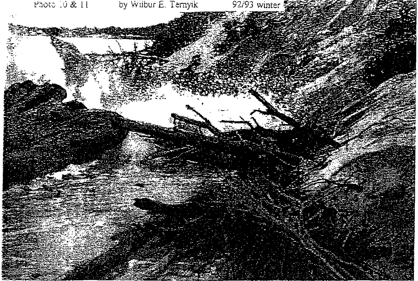
Location: Shelter Cove, north erosion area south end. Illustrating severe toe of the slope erosion caused by ocean wave surge.
